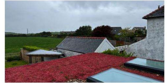
View: North West
